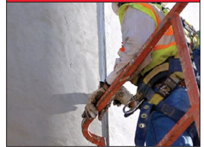
PRECAST WIND TURBINE TOWER
